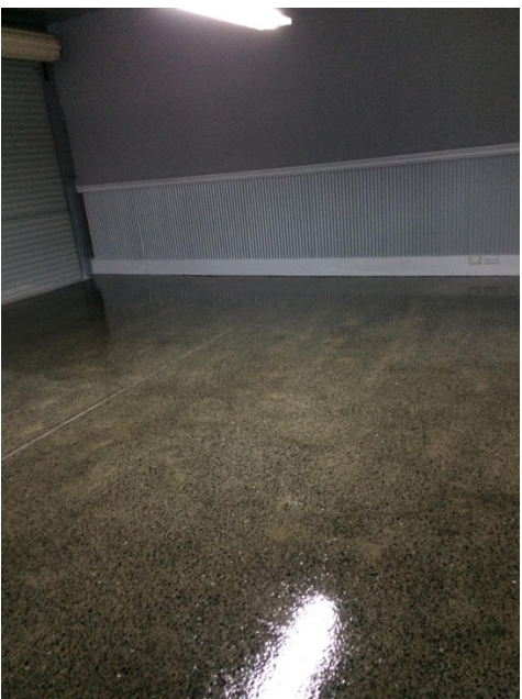
Figure 1 Clear coat floor sealant – 2 X coat roller application
