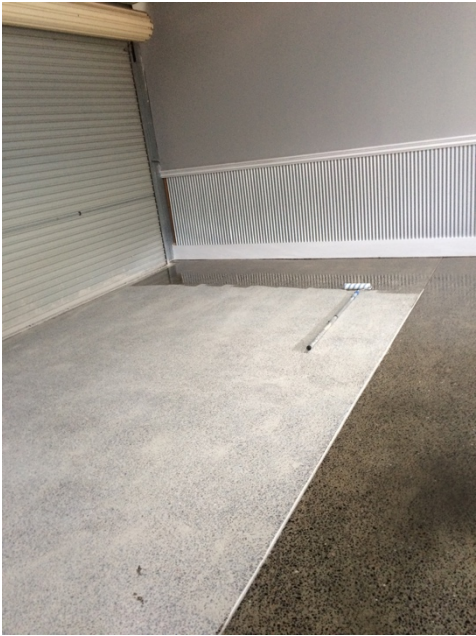
Figure 1 Clear coat floor sealant – 2 X coat roller application
